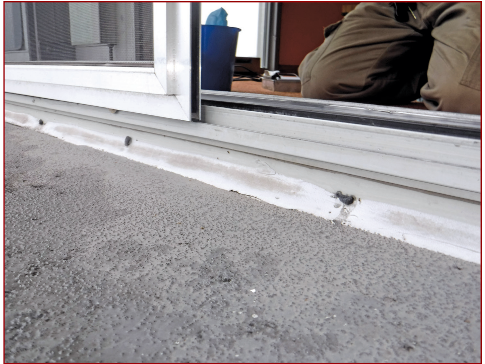
Figure 12 – Reticulated foam stuffed into weep ports of the terrace slider do more harm than good. Any porosity the material had is compromised by 1) forcing the material in a hole smaller than the piece of material that is intended to fill it and 2) the material fulfills the role of a clogged filter due to the abundance of silt in the subframe.
