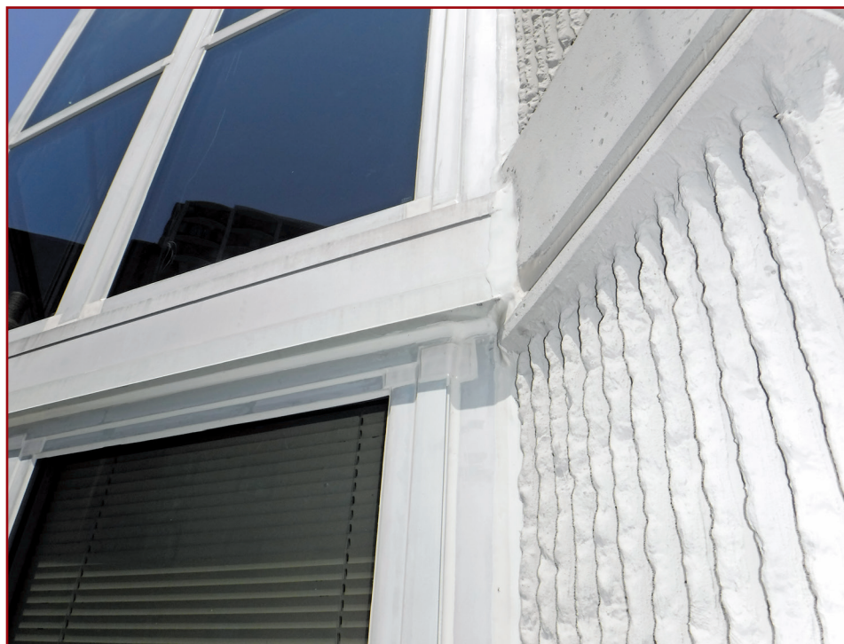
Figure 7 – Revised barrier system that places emphasis on a more targeted approach, resulting in a more aesthetically pleasing finished installation (cap beads, fillet beads, target patches).
