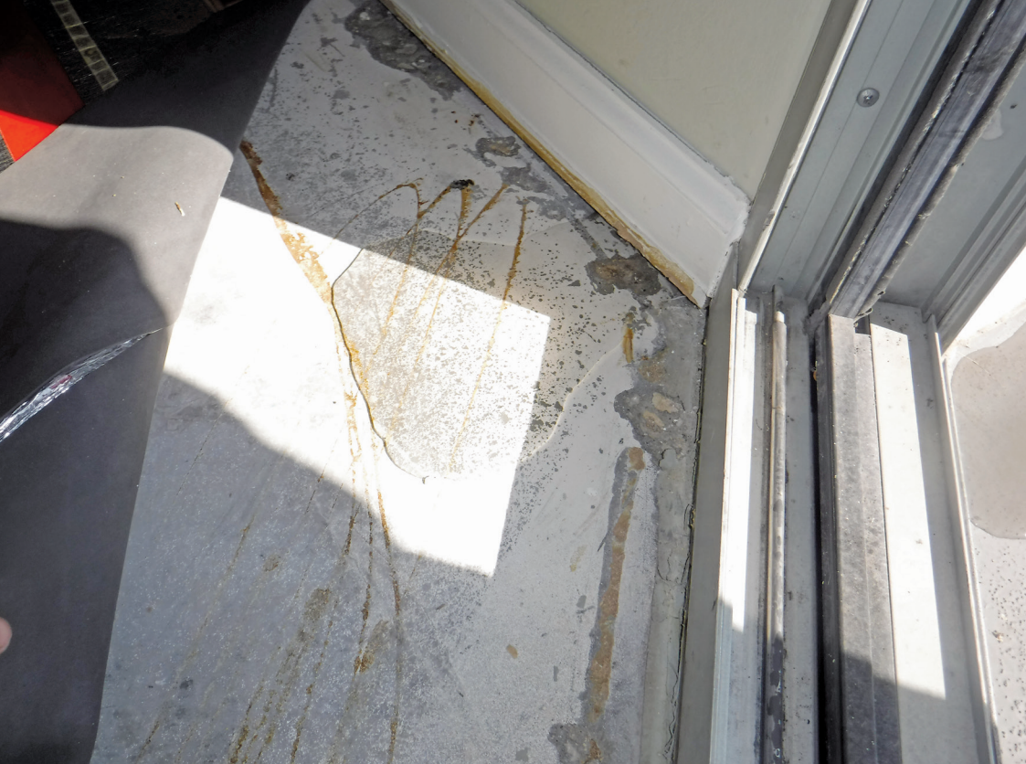
Figure 6 – Free moisture pooling on the interior of the occupancy adjacent to terrace sliding door. The source was confirmed as water that was introduced to the sill receptor via the weep structure of the hopper window, some 12 feet removed from this location.
