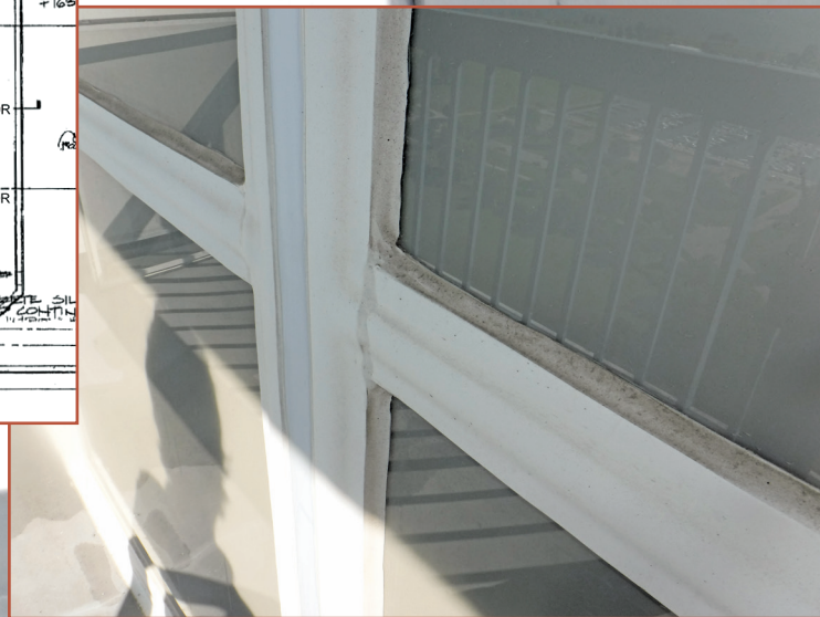
Figure 3 - The more aggressive barrier system compromised the overall aesthetics and was not well-received by unit owners.
