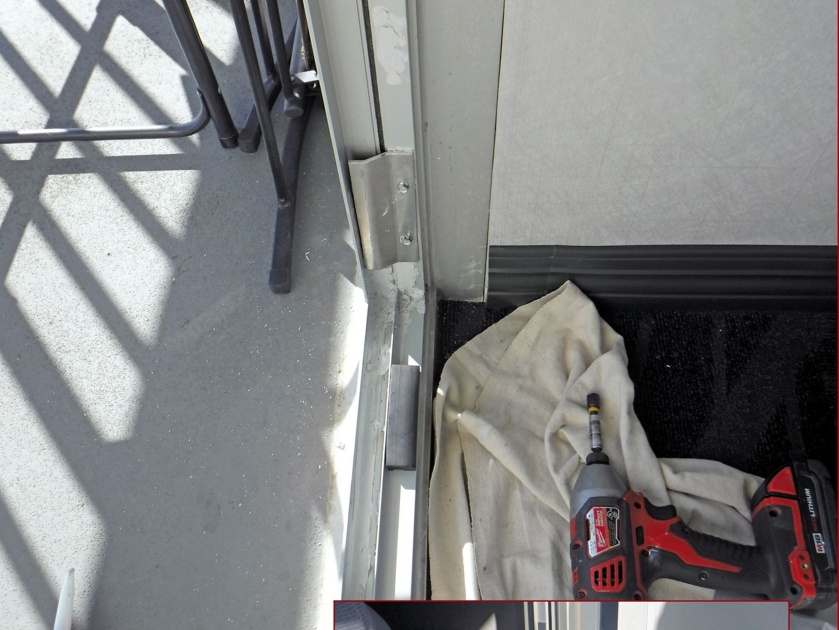
Figure 9 – During the dry fit process, shims in the sill are adjusted, and clips are installed in the jambs.
