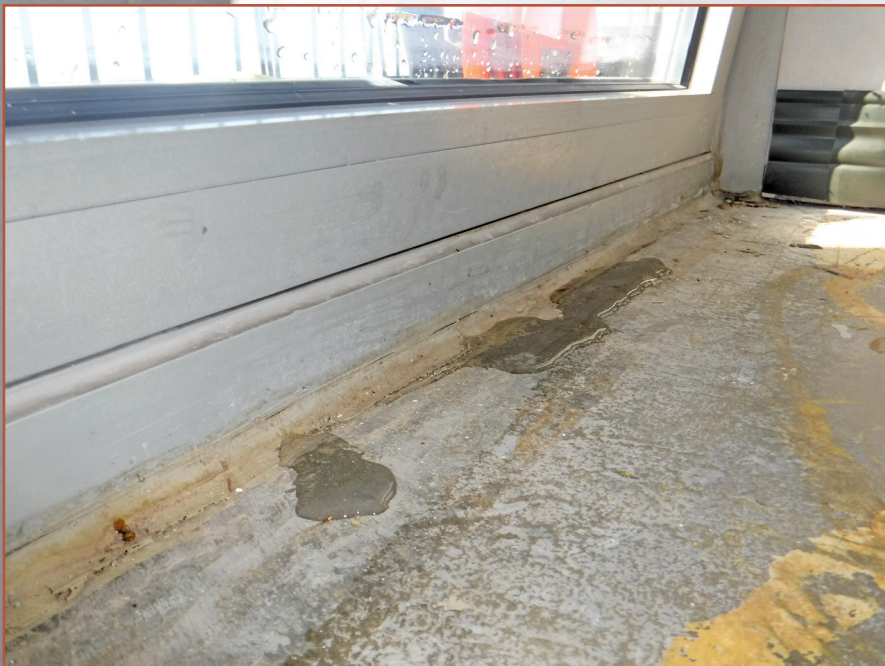
Figure 5 – Free moisture pooling on the floor interior after “static” water test (came in at localized areas of bond failure between the sill extrusion [receptor frame] and sealant joint).
