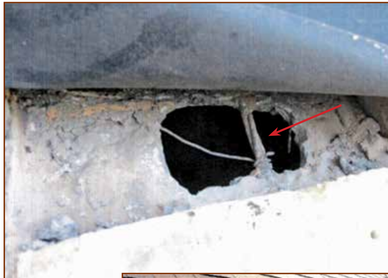
Photo 1 – Spiral-wound steel reinforcement of concrete deck.
