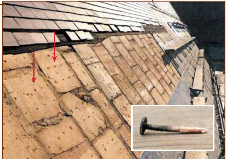
Photo 2 – Overall condition of structural clay tile roof deck with uniformly spaced rows of pockmarks from the original nailed installation of flat-slab clay tile.
