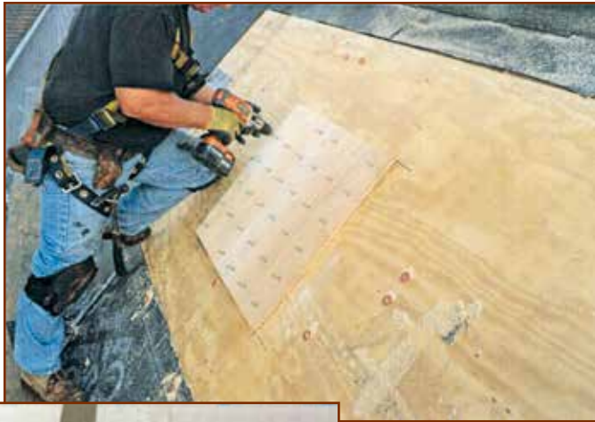
Photo 6 – Contractor preparing test panel for pull test under field conditions.
