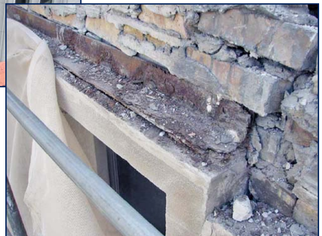
Photo 9 – Typical corrosion of loose steel lintels at window head of gable features.
