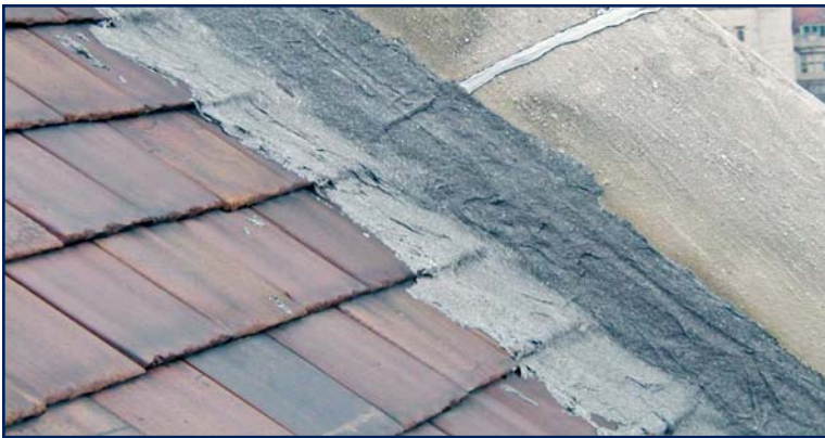
Photo 7 – Repeated applications of cold-process repairs at rakes with adjacent stone coping.
