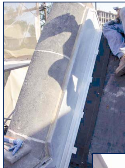
Photo 15 – Completely reinstalled stone coping with integrated through-wall and accessory counterflashing assembly ready for the installation of clay tile.
