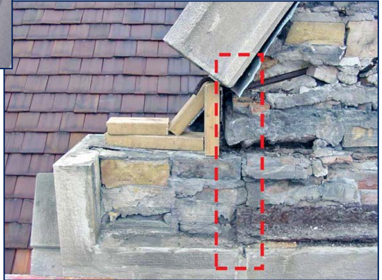
Photo 11 – Lack of continuity in through-wall flashing resulting in corrosion of loose steel lintel below.
