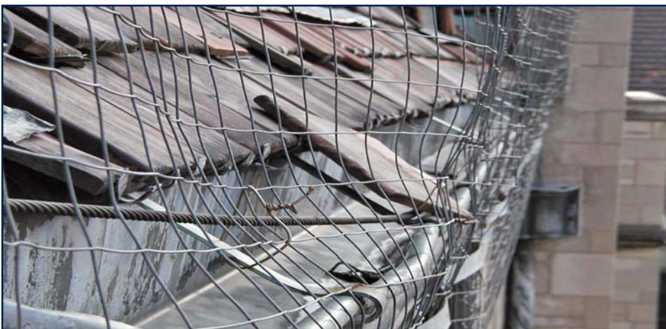
Photo 6 – Netting installed as emergency response to falling tile.
