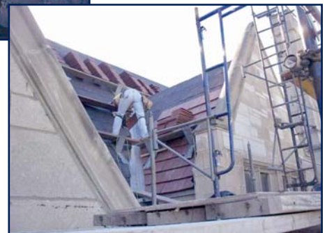
Photo 16 – Installation of clay tile subsequent to the completion of adjacent cladding repairs.
