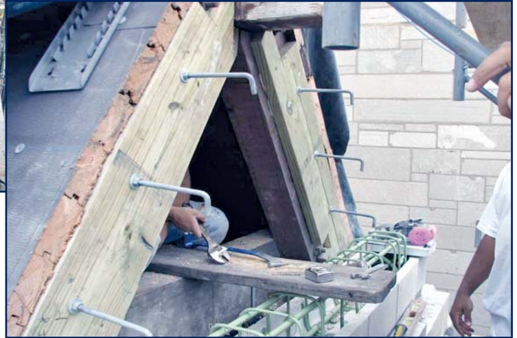
Photo 14 – Gable end rebuild with new bond beam and “J” hooks that will interface with fully grouted, steel-reinforced CMU backup wall.
