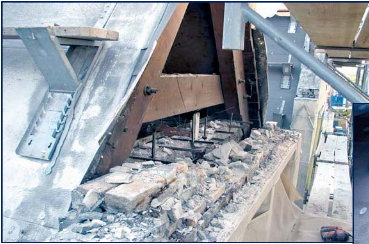
Photo 13 – General limits of demolition at gables with temporary roof covering established.
