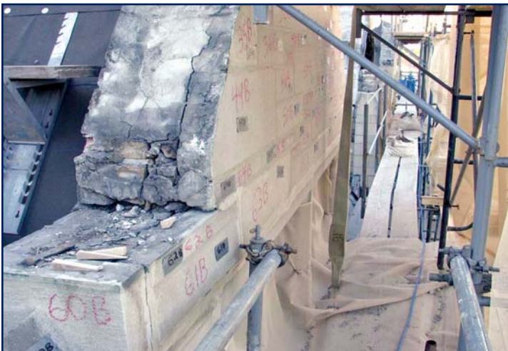
Photo 12 – Cataloguing of stone cladding ahead of required selective removals for the gable, backup wall rebuild.
