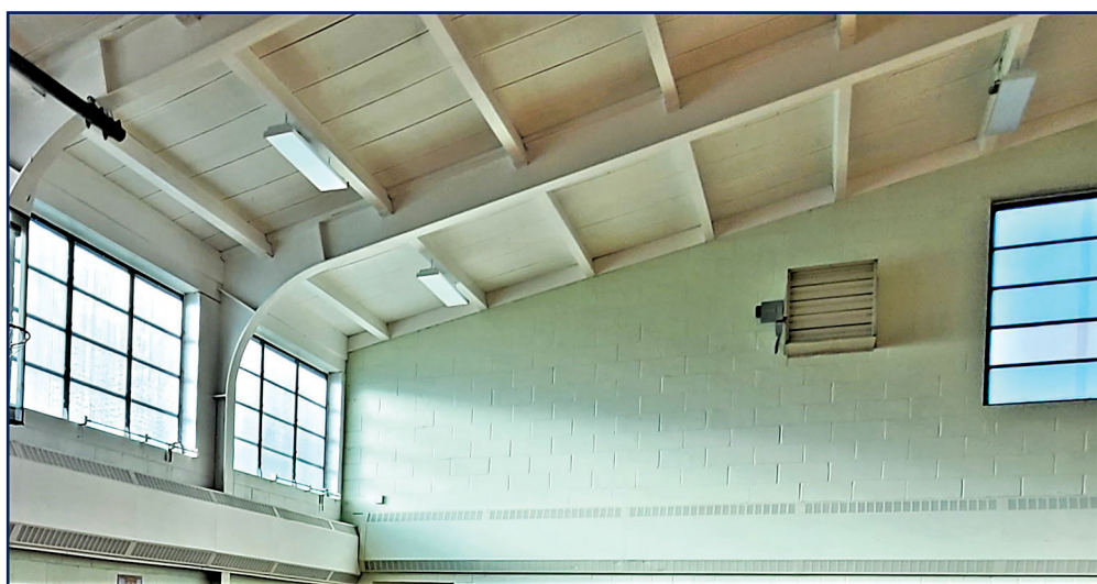
Figure 1. Somewhat obscure in terms of modern market share, structural fiberboard decks are more likely to be encountered on older buildings. This application involves tapered steel beams/columns forming a rather long-span occupancy. Image courtesy of William J. Hope, RBEC, RRC, RWC, REWC, RRO, PE, CCS, GRP, CSRP (Exterior Consulting and Roof Management, Albany, NY).
