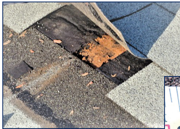
Figure 2. Marketed for both pitched and low-slope configurations, failure of the covering could compromise the planks. Here, shingles were used at a slope much too shallow for proper service, and the deck has suffered as a consequence. Image courtesy of William J. Hope.
