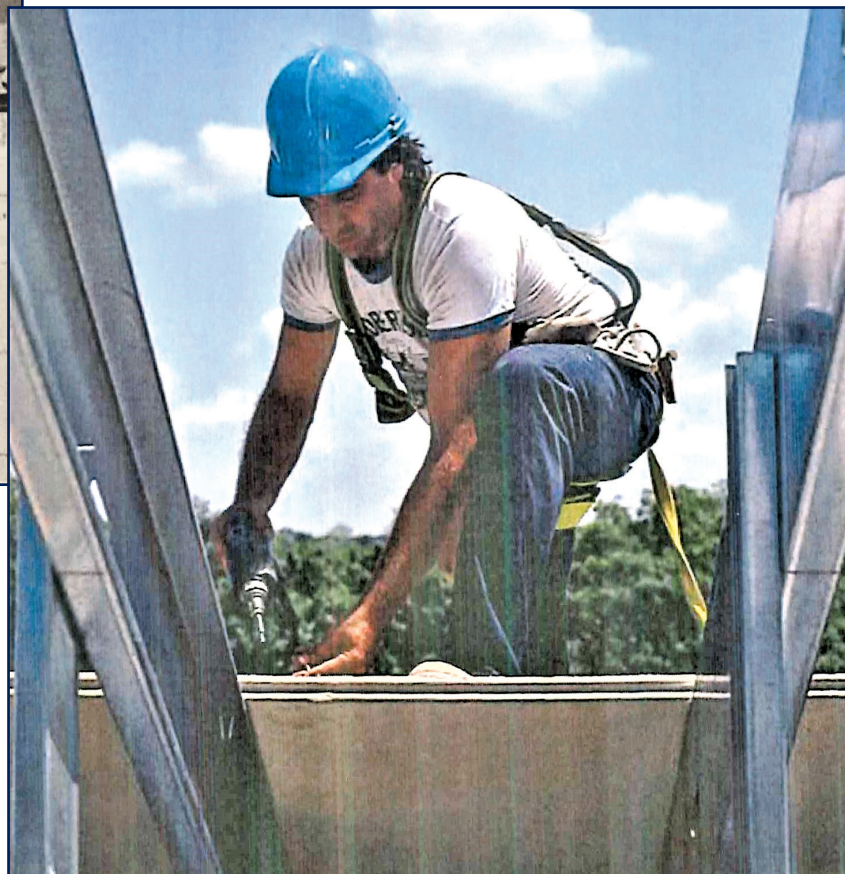
Figure 8. The product can be screwed down to metal framing elements. With appropriate fastening devices and tongue-and-groove edges advancing, the planks can serve as a shear diaphragm as well as substrate for the roof covering. Image by permission from Homasote Co.
