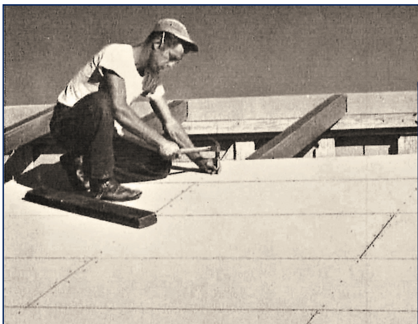
Figure 7. Manufacturers' recommendations state that butt-joints must occur on framing members. Beyond this, panel ends must not project beyond framing members at roof perimeters; that is, planks are not intended to be in an exposed-eave arrangement. Image by permission from Homasote Co. (Note: This photo was taken prior to current safety standards.)
