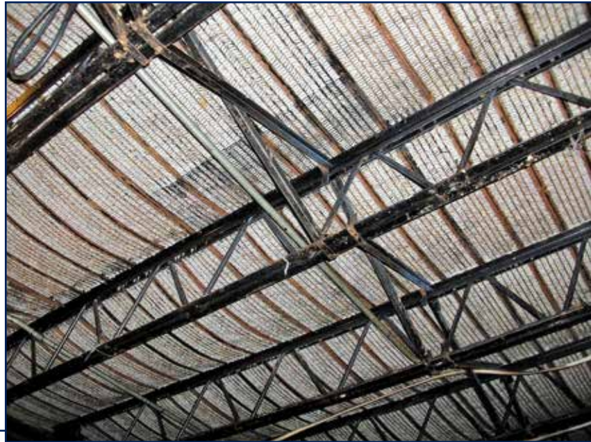
Figure 8 – Expanded wire lath was a common permanent form in decades past.
