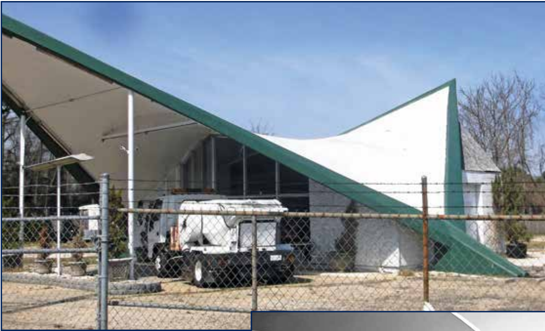
Figure 2 – Cast-in-place concrete may be configured to many different profiles. Here, the designer envisioned a hyperbolic paraboloid saddle.
