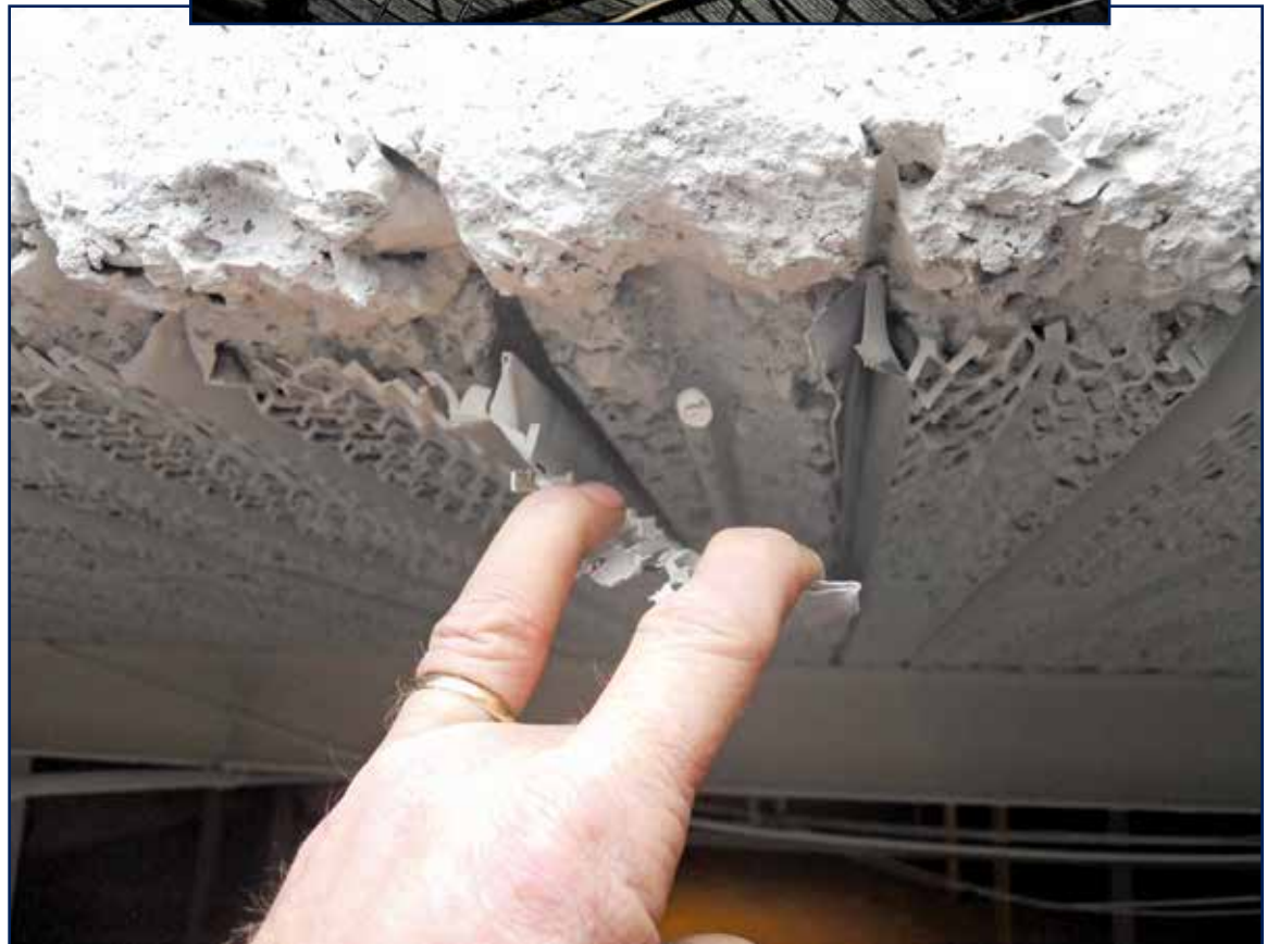
Figure 9 – Cinder concrete atop expanded wire lath (image courtesy of Donald Kilpatrick).
