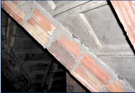
Figure 3 – Clay tile units mortared into place as fire-safing over structural steel in an old attic.
