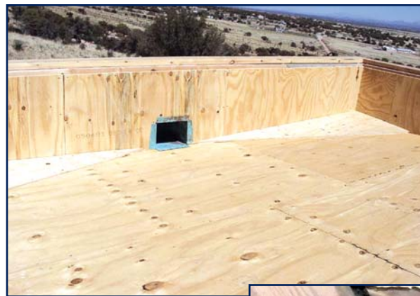
Figure 9 – Crickets/saddles can be crafted with plywood to effectively divert water.
