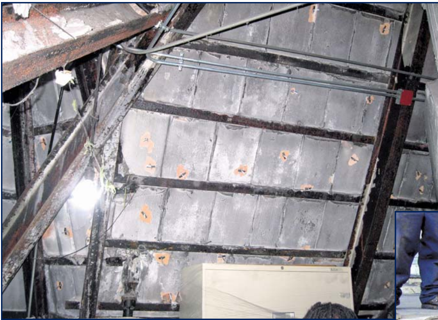
Figure 7 – Attachment of new plywood cladding using toggle bolts.
