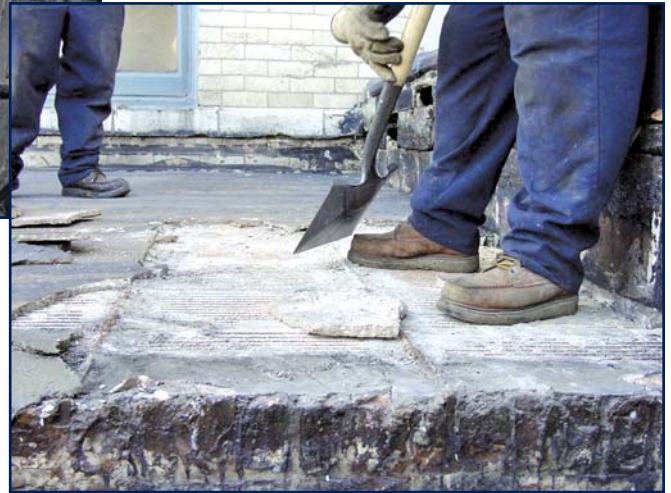
Figure 8 – Delamination and spalling of mortar topping course.
