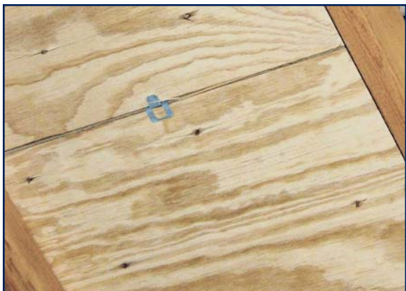
Figure 12 – H-clips (panel edge clips) reduce the effective spacing of framing members, better distributing loads to adjacent panels.
