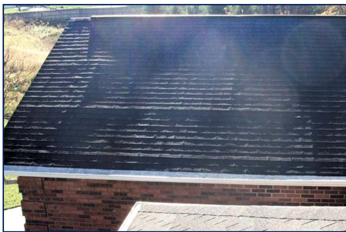
Figure 11 – Deck buckling from substandard ventilation, improper attachment along panel edges, or failure to provide space between sheets.
