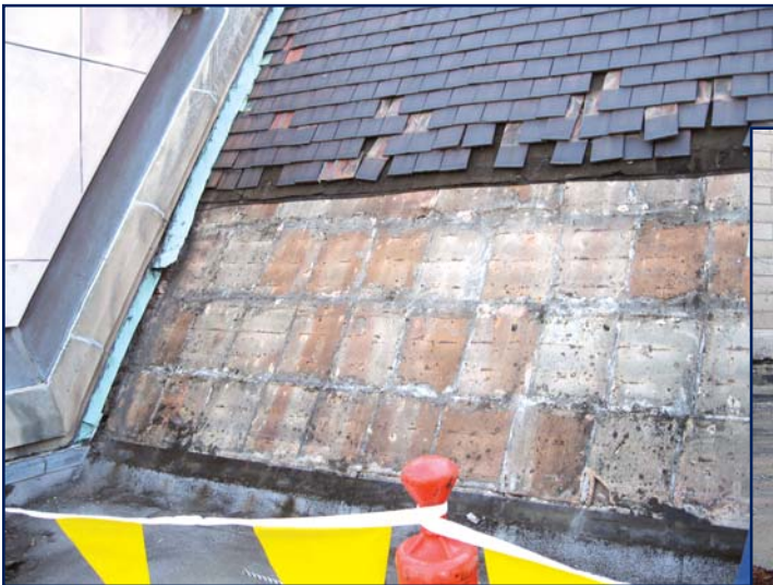
Figure 5 – Tile covering on clay tile deck on a vintage pitched roof.
