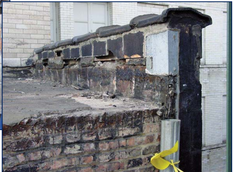
Figure 6 – Tiles cast into the inboard face of a parapet.
