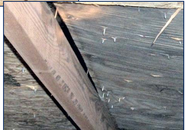
Figure 10 – Permanent distortion from insufficient fastening along edges, likely aggravated by substandard attic ventilation.
