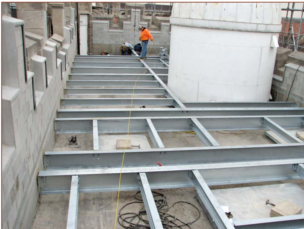
Photo 9 – The introduction of new, galvanized structural framing elements above the original roofline.
