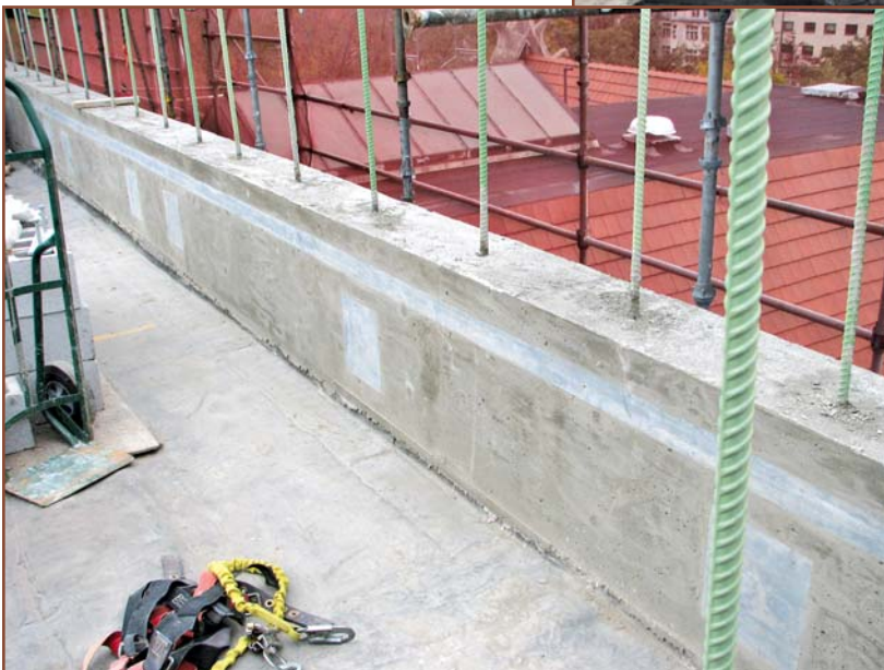
Photo 5 – Forms stripped, exposing interior face of new concrete beam fitted with embedded weldments.
