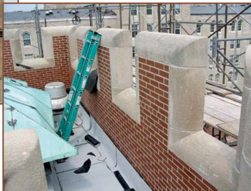
Photos 1A and 1B – Examples of a "crenellated" parapet wall or battlement as identified by the alternating high (merlon) and low (crenel) points of the feature.
