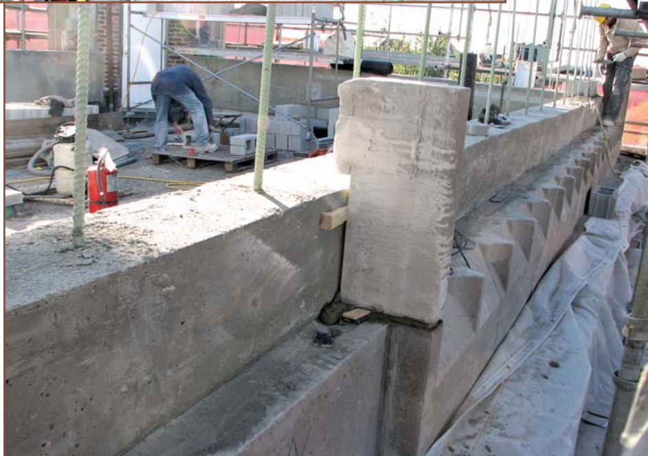
Photo 6 – Stone requiring field cut to accommodate new tolerances established by the concrete beam.
