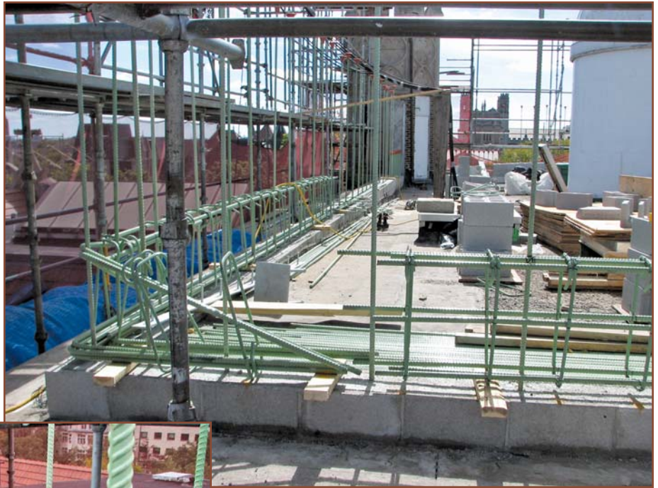
Photo 4 – Rebar set for forming and pouring of a new concrete beam above existing roofline.
