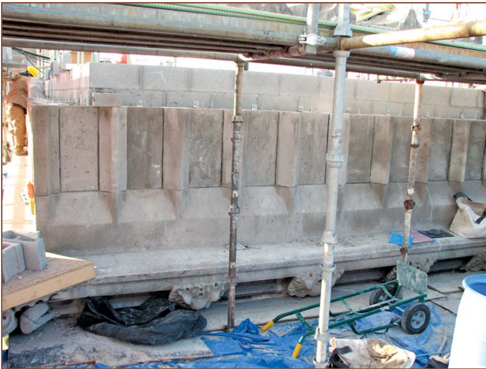
Photo 7 – Reinstallation of cut/carved limestone cladding with stainless steel anchors.
