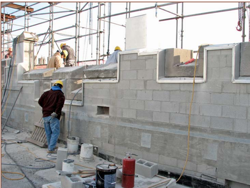
Photo 8 – Fully integrated zinc- and tin-coated copper receiver flashings below stone copings.
