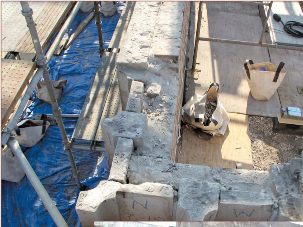
Photo 2 – Cut/carved stones labeled for correct spotting during reconstruction.
