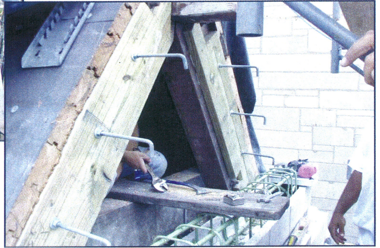
Photo 14 – Gable end rebuild with new bond beam and “J” hooks that will interface with fully grouted, steel-reinforced CMU backup wall.
