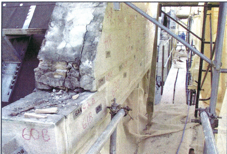
Photo 12 – Cataloguing of stone cladding ahead of required selective removals for the gable, backup wall rebuild.
