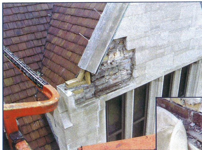
Photo 8 – Inspection opening at area of localized distress at gables.
