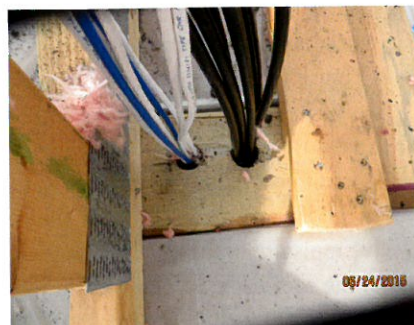
Photo #4 – Vapor retarder bypass through top plate of partition wall.
