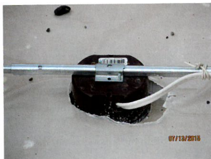
Photo #3 – Vapor retarder bypass at ceiling light electrical box.
