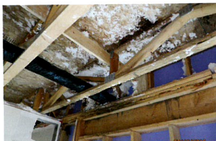
Photo #5 – Leaky dryer and bathroom vent ducts in truss space.
