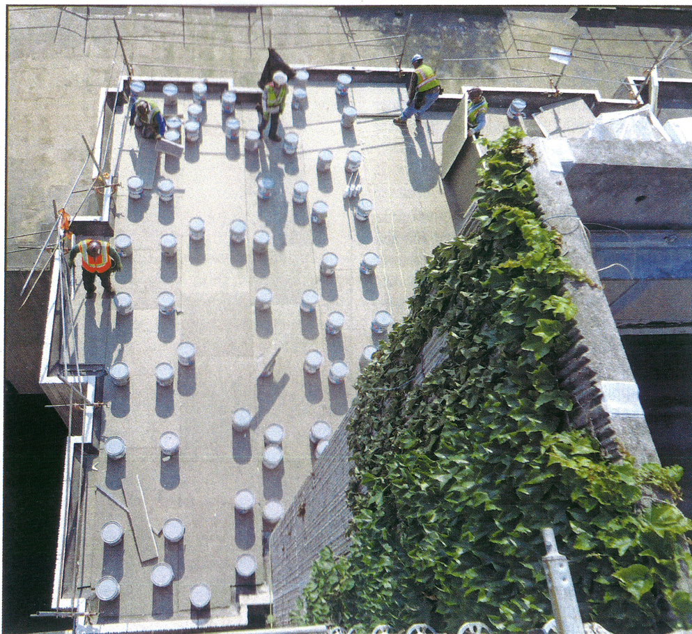
Photo 1 – Contractor using pails of materials that have exceeded their shelf life as temporary ballast on a low-rise foam installation.
