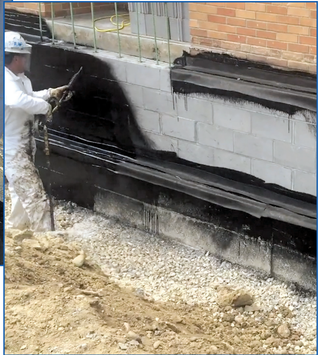
Figure 3. Vertical spray application of polymer-gel waterproofing system.
