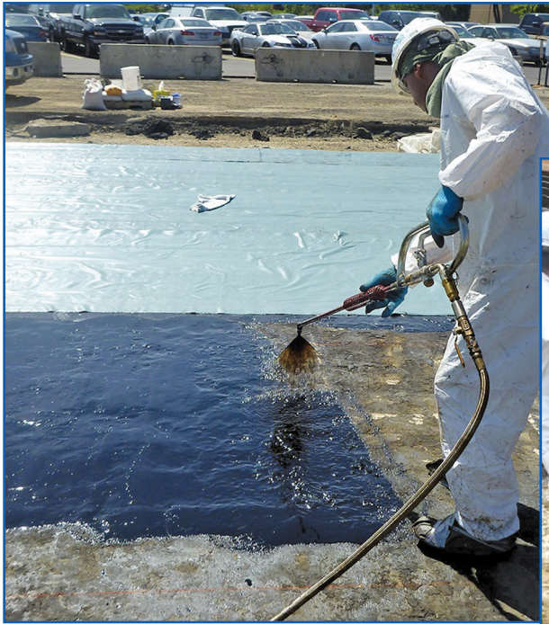
Figure 2. An example of horizontal spray application of polymer-gel waterproofing system.
