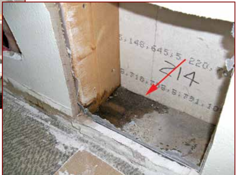
Photo 2 – Re-created water intrusion into wall system.
