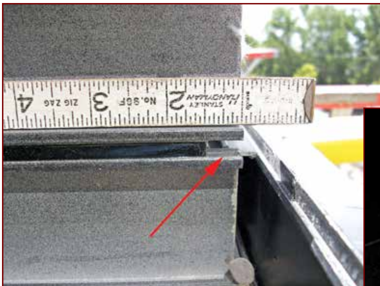
Photo 3 – The window thermal break had shrunk ½ in.
