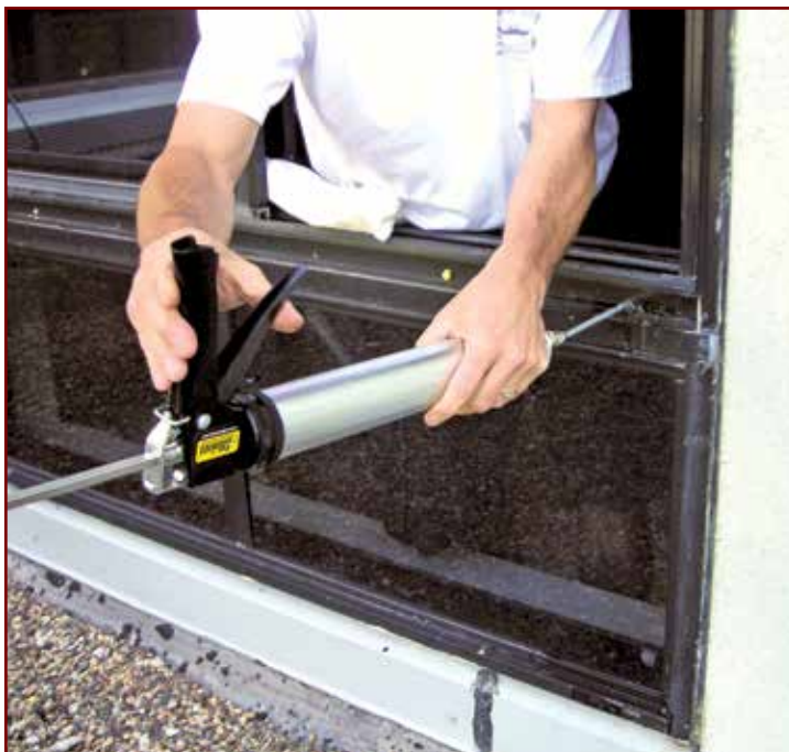
Photo 7 – The hydrophilic grout is injected.
