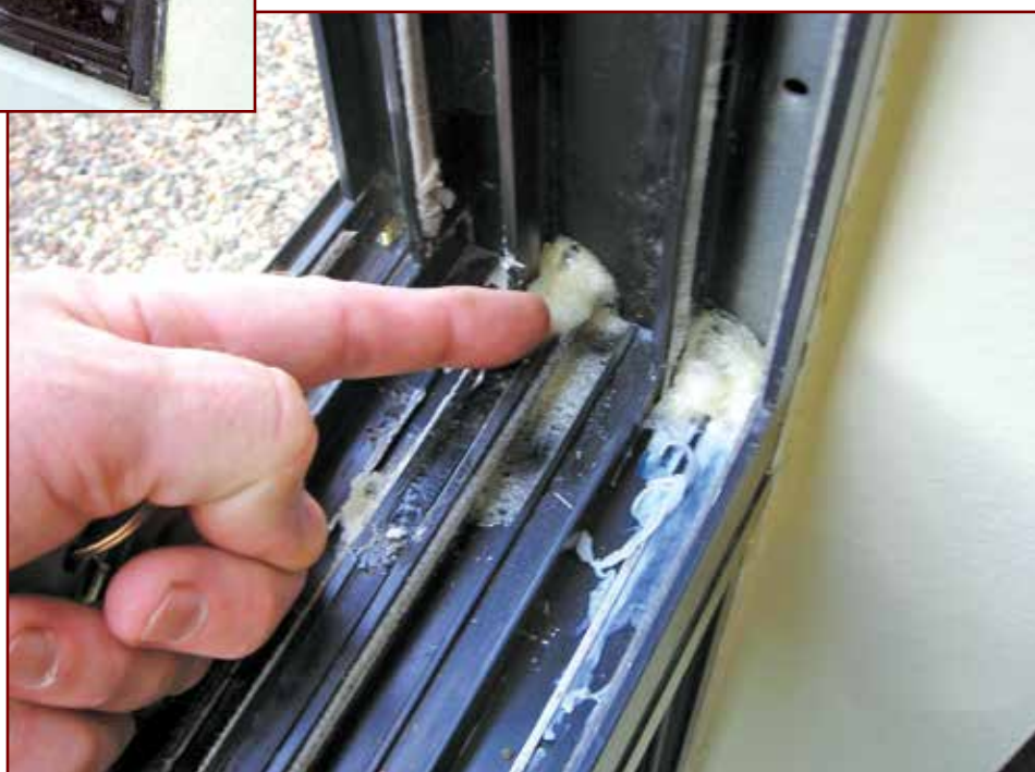
Photo 8 – Grout foaming up through existing weep holes indicating a complete seal at window jamb.
