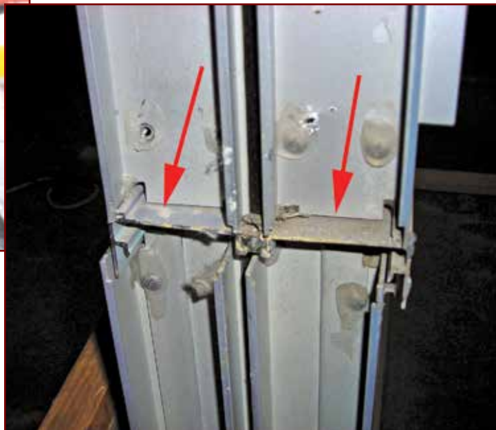
Photo 4 – Silicone sealant missing.
