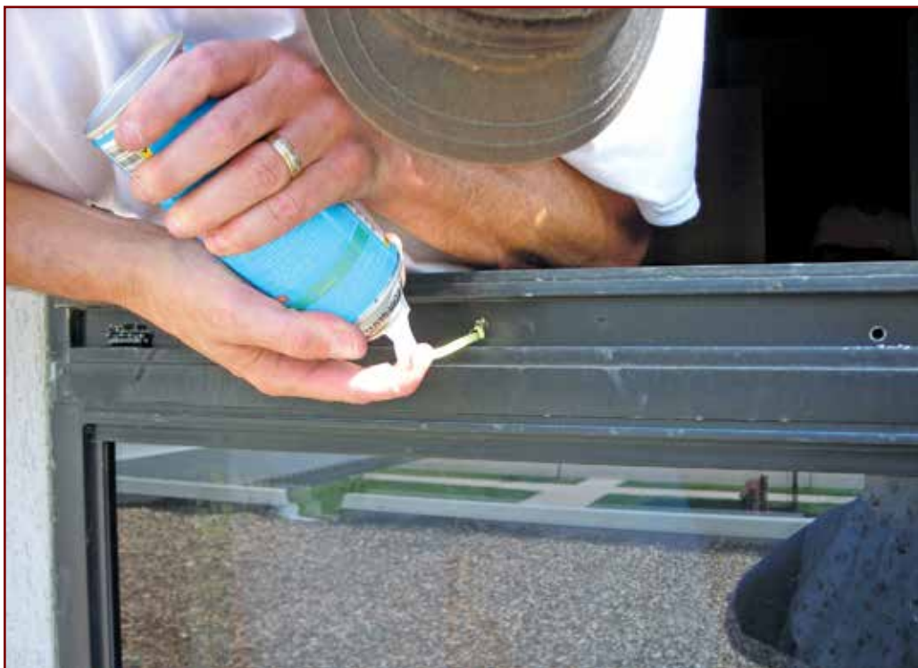
Photo 6 – The “containment dam” foam is injected.
