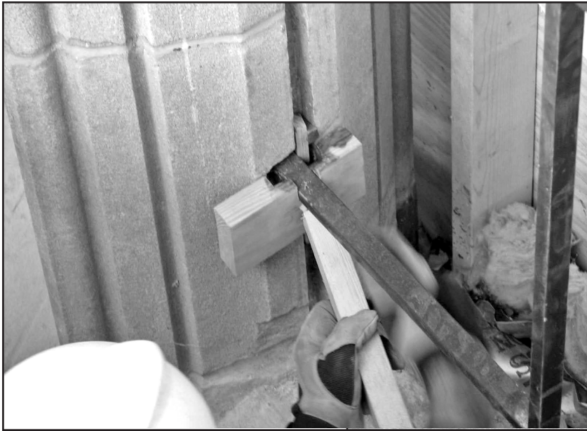
Photo 13 – Wood forms set in advance of pouring molten lead to fill the pocket in the stone surround.
