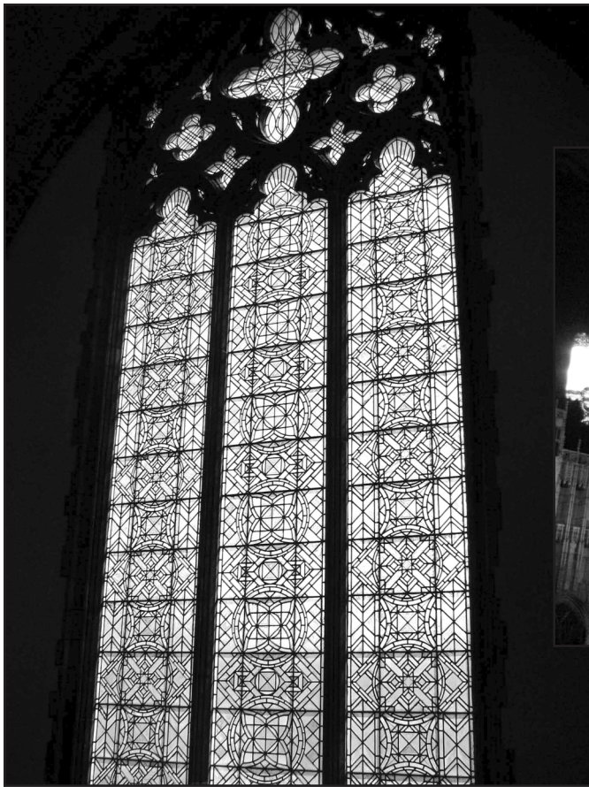
Photo 3 – Typical lancet window as seen from nave interior.
