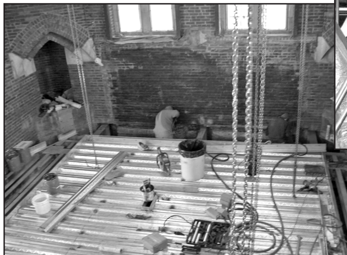
Photo 20 - Ironworkers setting new steel framing and decking for the playing cabin at the 160-ft level of the tower interior.
