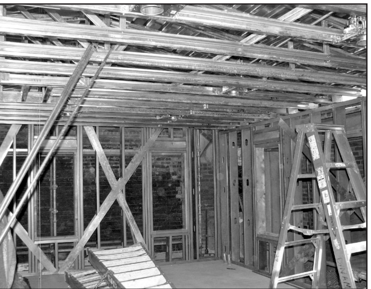
Photo 21 - New wall framing and truss assembly for the playing cabin.
