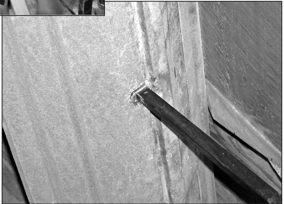
Photo 14 – Finished interface of exterior support bar framing and stone surround.
