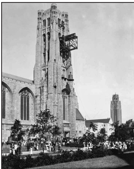
Photo 5 – Circa 1934 loading of the tower with carillon bells.
