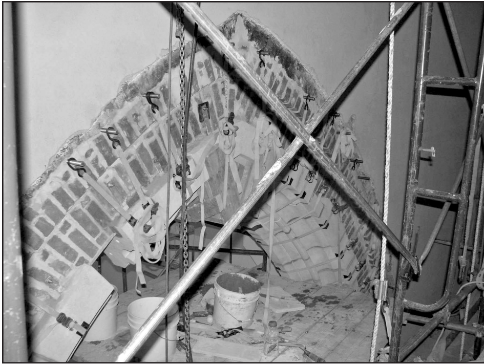
Photo 16 – Final setting of cut limestone surround in tonal opening.
