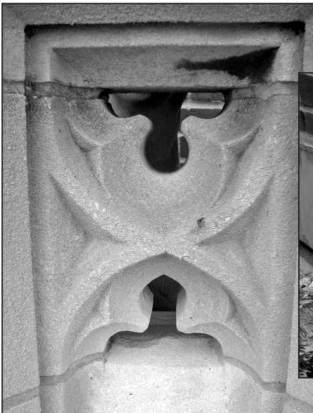
Photo 10 - Carved stone central to the three-stone set establishing the portal openings.
