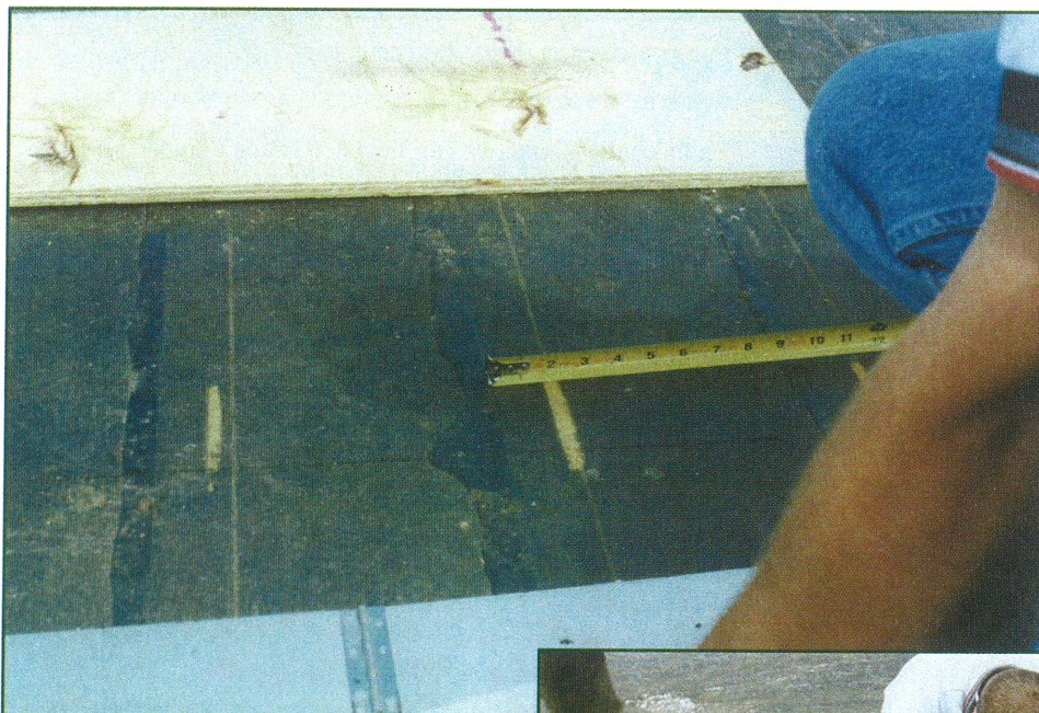
Photo 4: Measuring felt ply headlap in pre-determined sample area.
