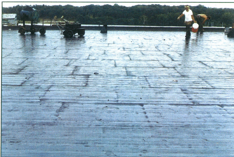
Photo 6: Results that can be anticipated when application temperatures are well above the product's EVT. Note the "picture framing" as a result of excessive temperatures and bleed-through at joints in the insulation.
