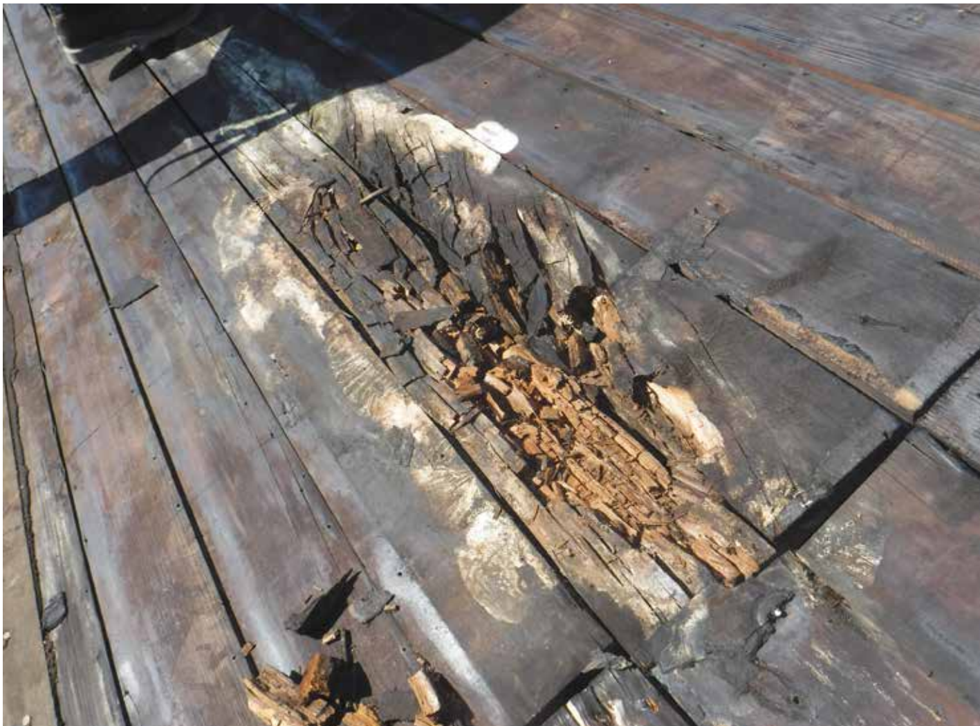
Figure 13. Inspection and identification of bad decking (2.5 in. thick and 5.5 in. wide tongue and groove) was performed topside after the removal of the existing standing-seam roof, insulation, and underlayment.
