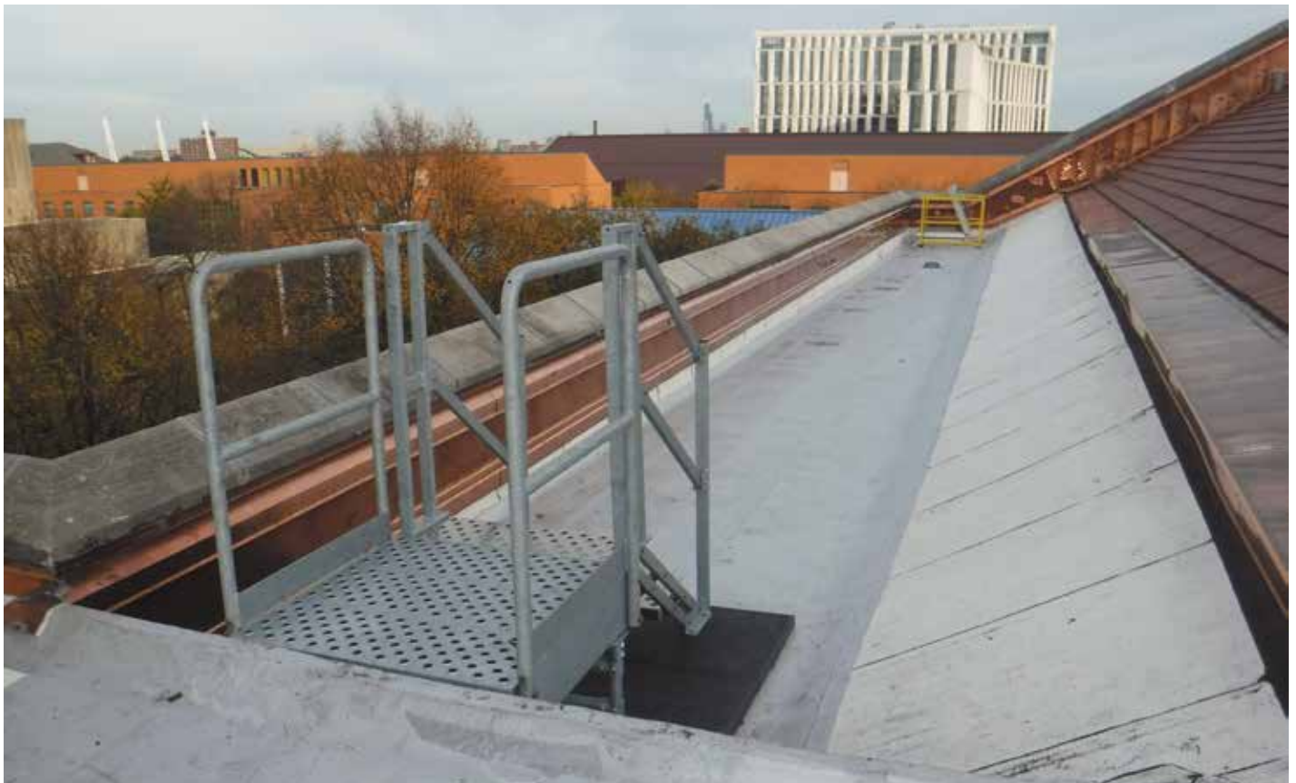
Figure 10. Overall completed northwest integral gutter drainage zone.
