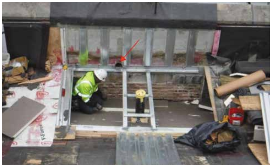
Figure 9. Crew installing the structural steel framing intended to carry the new galvanized decking and hat channels on the roof side of the parapet wall that is the receiving substrate for the plywood sheathing, establishing the substrate for the new flat-lock-seam copper panels. The existing through-wall drain will be closed off and the new parapet wall section will be cored through, establishing provisions for overflow drainage for each of the four roof drainage zones.
