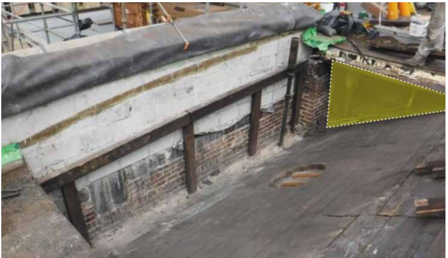
Figure 11. Typical condition as encountered in each of the four integral gutters. See Fig. 9 and 12 for additional information related to new design intent and solution for venting of the triangulated, “dead” air space that will be maintained as part of the new as-built condition. New insulation was required from the interface of the parapet wall upslope to the skylight curb.
