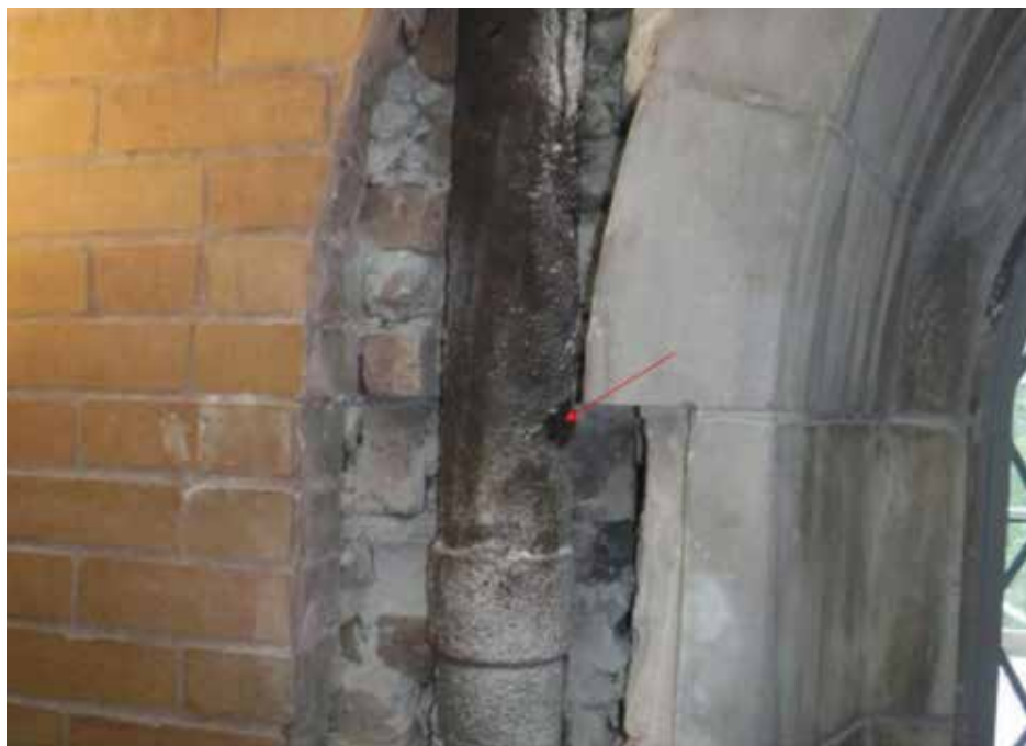
Figure 6. Original drain riser buried in the mass wall. Corrosion of the piping resulted in damage to the stone surrounding the adjacent window opening.
