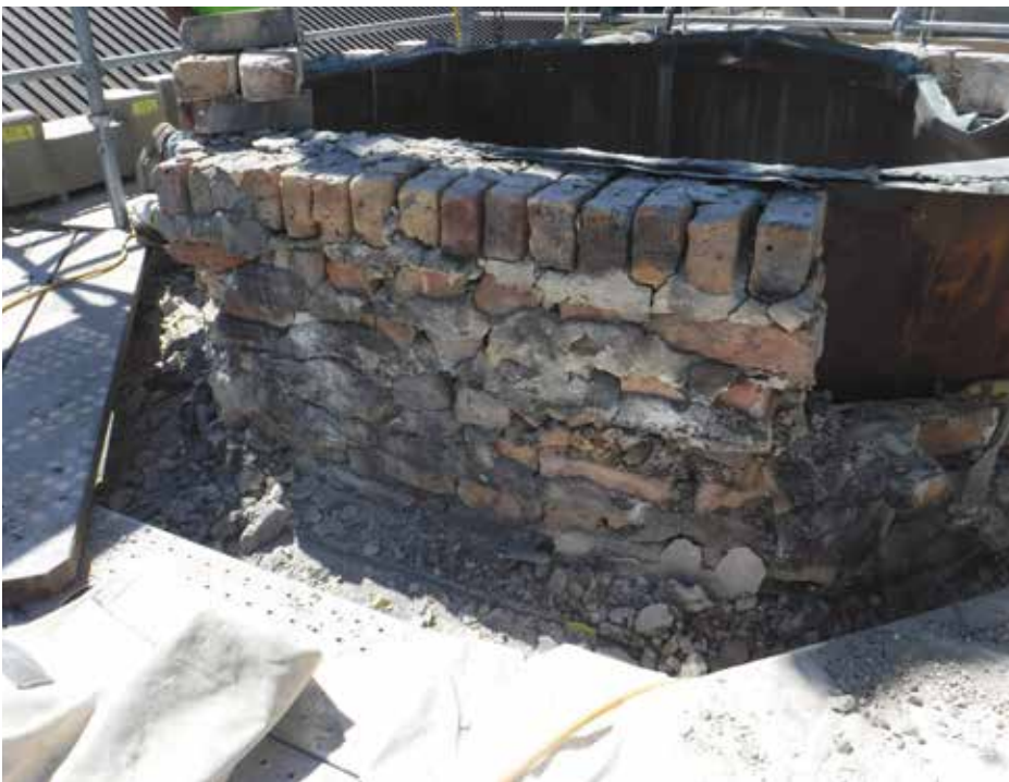
Figure 4. Overall poor condition of existing brick masonry backup wall found to be typical on each of the four turrets.
