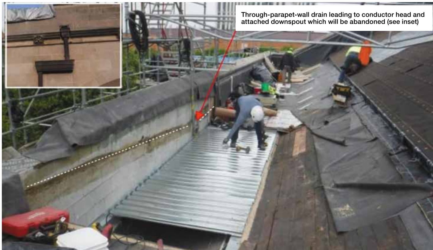
Figure 7. The introduction of new galvanized steel roof deck and framing members into one of the four primary drainage zones. The line on the back side of the new steel-reinforced, grouted concrete masonry unit backup wall represents the location of the slope to drain feature that was accommodated by the wood cribbing that was original to the building. A fully tapered insulation atop the new steel deck will move water to the new drains at new locations (see Fig. 5).
