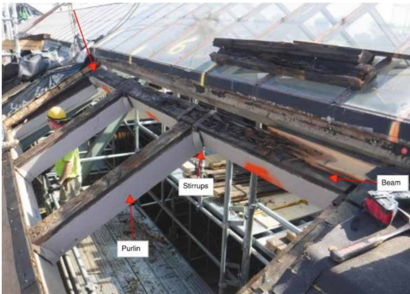
Figure 14. Decking removed, exposing water-damaged timber beam framing at base of original skylight curb. The beams ran north-south, intersecting with east-west purlin at regular intervals between the steel trusses. The purlin had to be removed to facilitate the replacement of the north-south beam.
