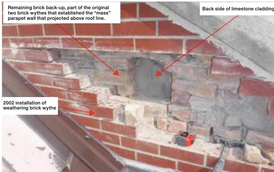
Figure 3. Through targeted removals it was determined that the exposed brick installed in 2002 as part of the conversion from field house to food services did not include brick ties. In addition, the bedding mortar that was present in the remaining wythe of brick (Chicago pinks) between the weathering wythe and stone cladding on the outboard side of the parapet wall had reverted to sand. A pocketknife could be used to pull brick from that area of the wall.
