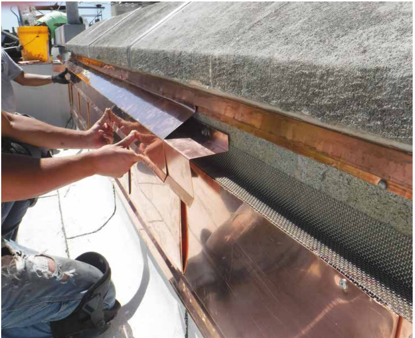
Figure 12. First in-place work of vented parapet wall assembly, including stainless steel insect screen and 32 oz copper hook strip for cap/counterflashing, providing a continuum of protection from above receiver for the through-wall flashing.
