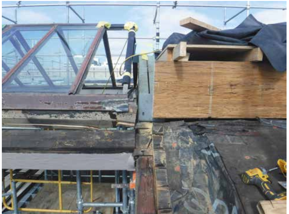
Figure 8. Original 1901 skylight curb on the left side with new curb on the right. Increased height was required to accommodate increased insulation thicknesses.
