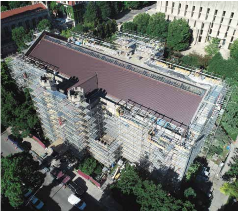
Figure 1. In September 2022, the building was fitted with scaffolding, hoisting bays, and monorails prior to roof and skylight replacement work scopes.
