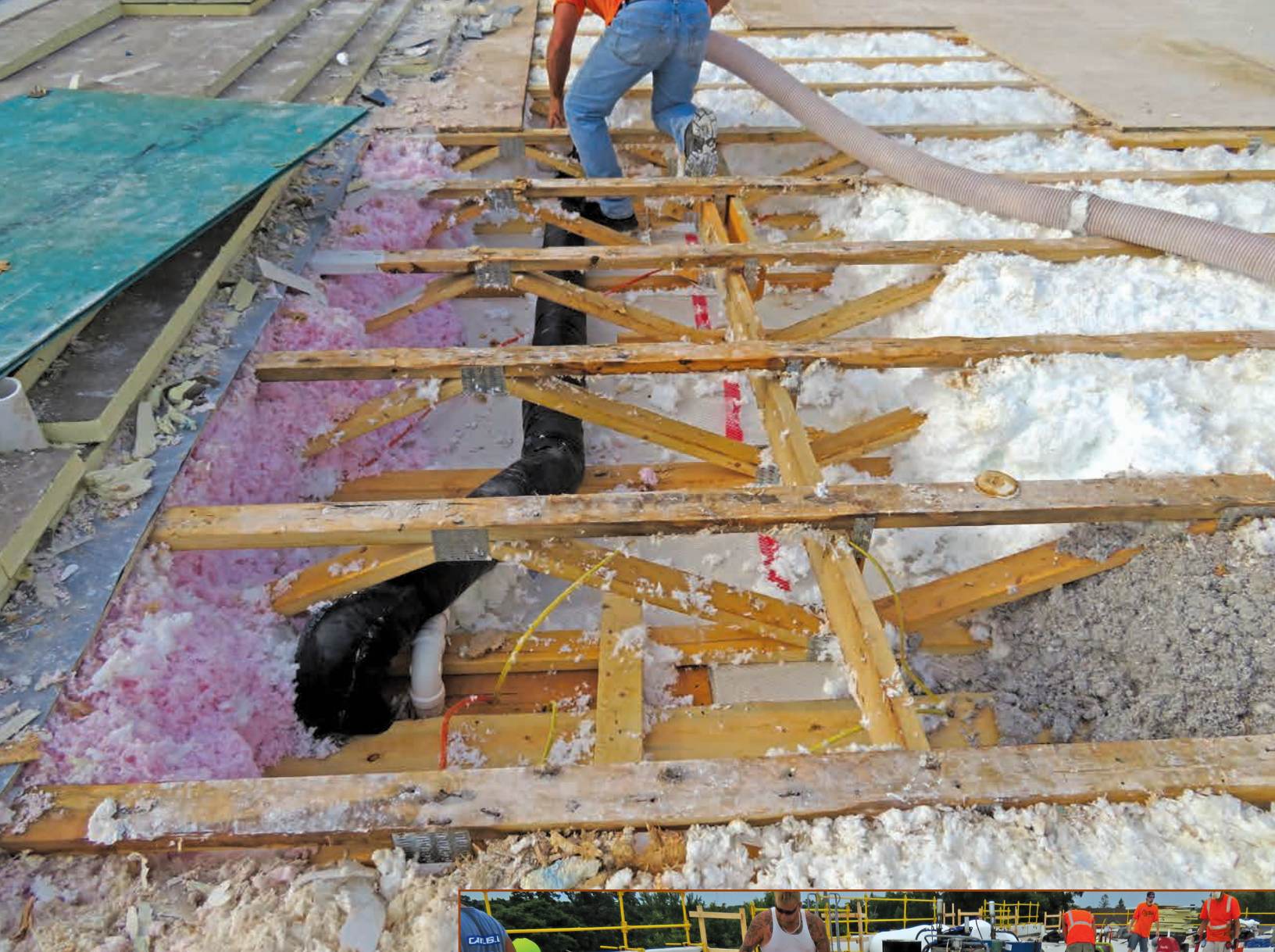
Figure 13 – Blown-in insulation.
