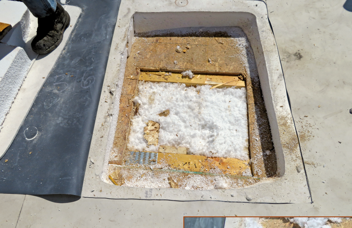
Figure 4 – Typical invasive inspection opening above trusses.
