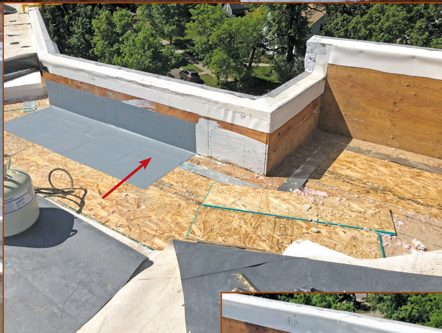
Figure 10 – Roof vapor/air barrier at roof perimeter.
