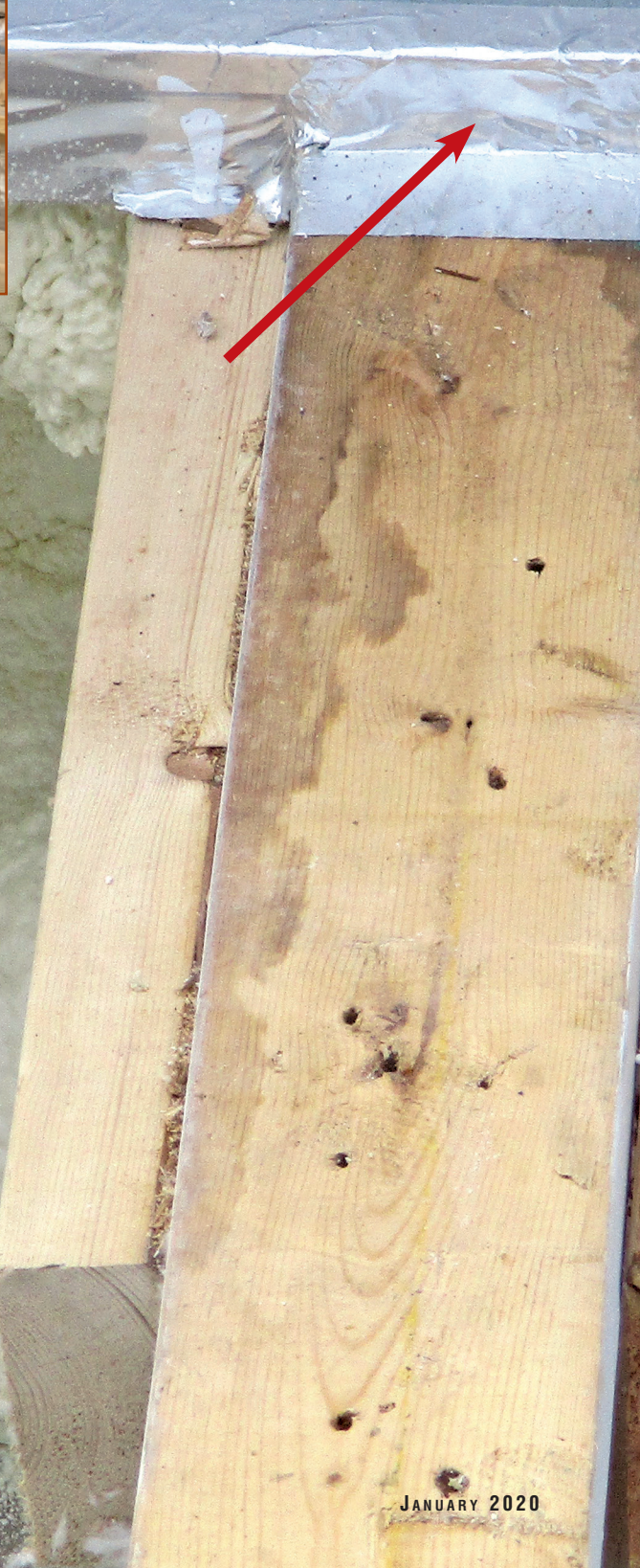
Figure 9 – Two-piece U-shaped vapor/air barrier transition metal.
