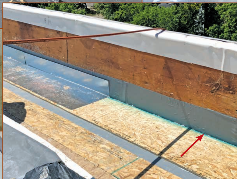
Figure 11 – Plywood and sheet metal angle parapet reinforcement.
