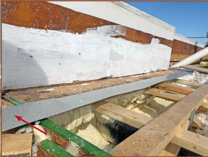
Figure 8 – Z-shaped vapor/air barrier transition metal.
