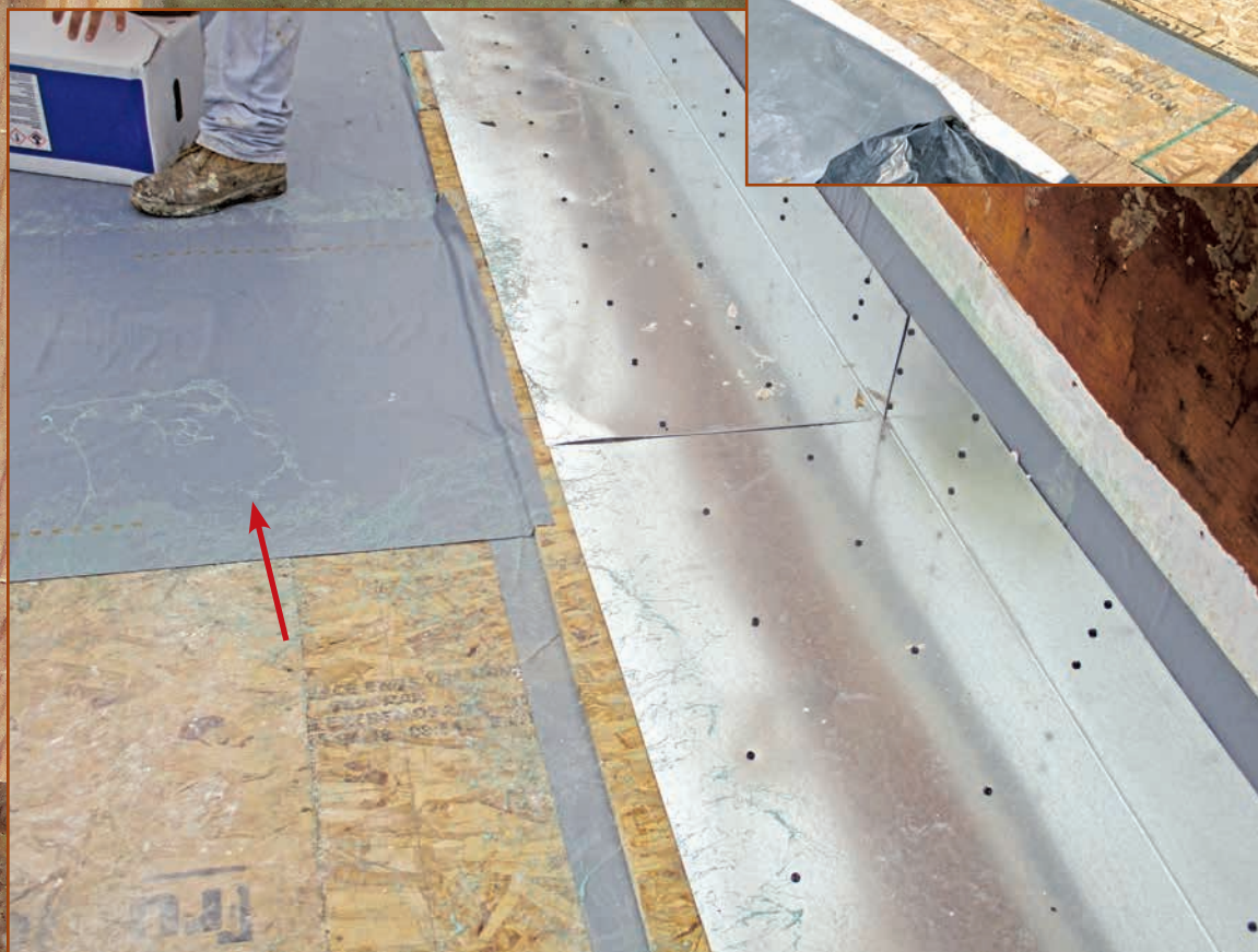
Figure 12 – Vapor/air barrier applied to field of roof.
