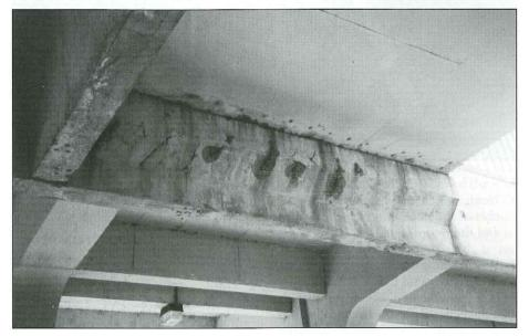
directly above the mark or, on the other hand, it could be caused by water leaking through the clamp ring of a plaza drain 10 feet away and following the underside of the sloped leader until it encounters a fitting, drops and stains the tile.
