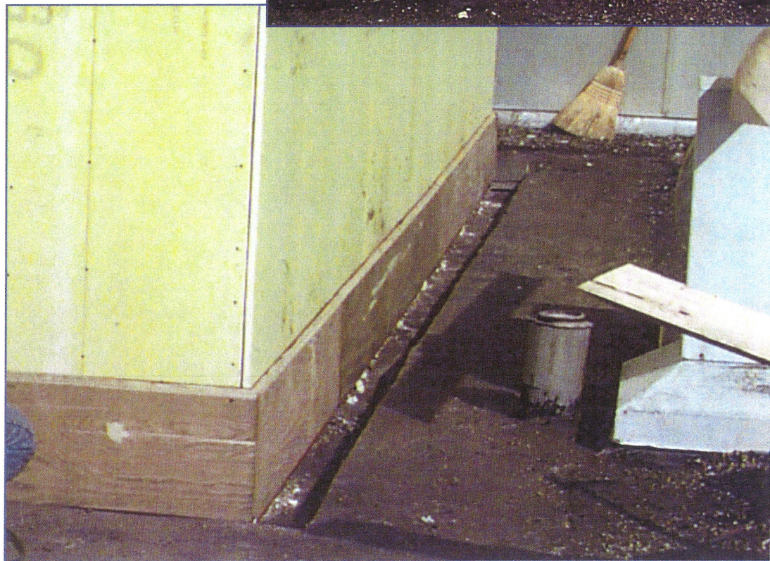
Below: Revised proper flashing conditions with required wood blocking.
