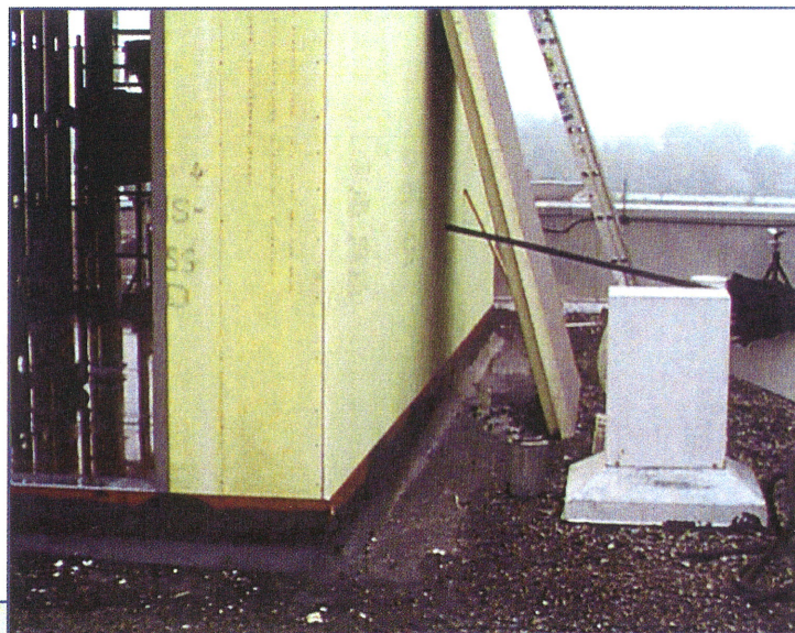
Right: Flashing of existing roof to steel curb.
