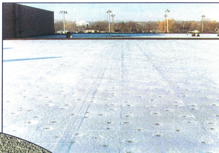
Above: The fastener pattern and frequency are demonstrated by heat loss in the frost on this adhered EPDM.
